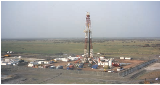
Operational conditions at the Thar Jath rig site.
