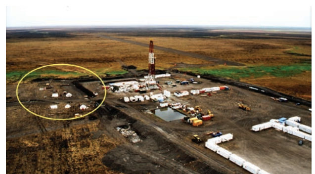
The Thar Jath site in April 1999. Security personnel lodged next to the camp indicated by a yellow circle.
